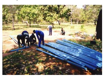
Fig. 6. Installation in a 130 m deep borehole with a water level of 90 m deep; the PVC pipes continue until the bottom of the borehole.
